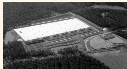
Our new distribution center in Windsor, Virginia.
